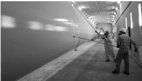
图 13 风机叶片喷涂过程 Fig.13 Wind turbine blade spraying process
